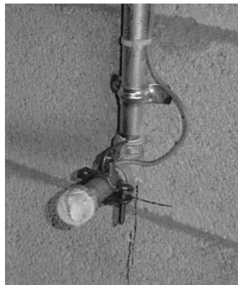
Figure 1 - Bond Clamp on Rigid Pipe
